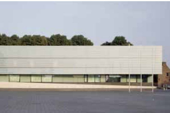
UN Studio's Het Valkhof Museum in Nijmegen, The Netherlands, uses translucent glass to diffuse light to the interior, which also reduces dangerous reflections. Photo courtesy of UN Studio.
