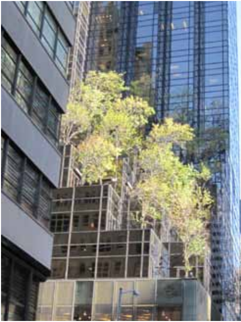
Plantings on setbacks and rooftops can attract birds to glass they might otherwise avoid. Photo: Christine Sheppard, ABC
