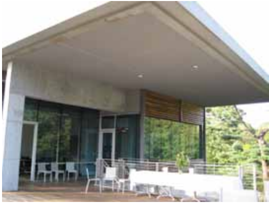
Overhangs block viewing of glass from some angles, but do not necessarily eliminate reflections. Photo: Christine Sheppard, ABC
