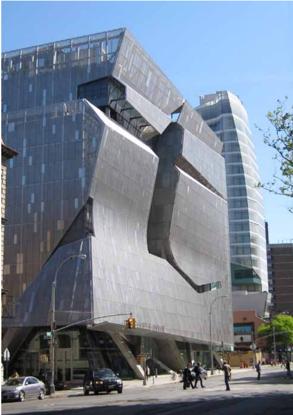
41 Cooper Square in New York City, by Morphosis Architects, features a skin of perforated steel panels fronting a glass/aluminum window wall. The panels reduce heat gain in summer and add insulation in winter while also making the building safer for birds. Photo: Christine Sheppard, ABC
