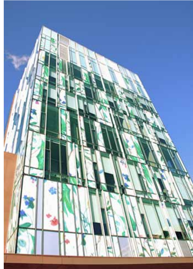
Issues of cost prompted Hariri Pontarini Architects, in a joint venture with Robbie/Young + Wright Architects, to revise a planned glass and limestone façade on the School of Pharmacy building at the University of Waterloo, Canada. The new design incorporates watercolors of medicinal plants as photo murals. Photo: Anne H. Cheung
