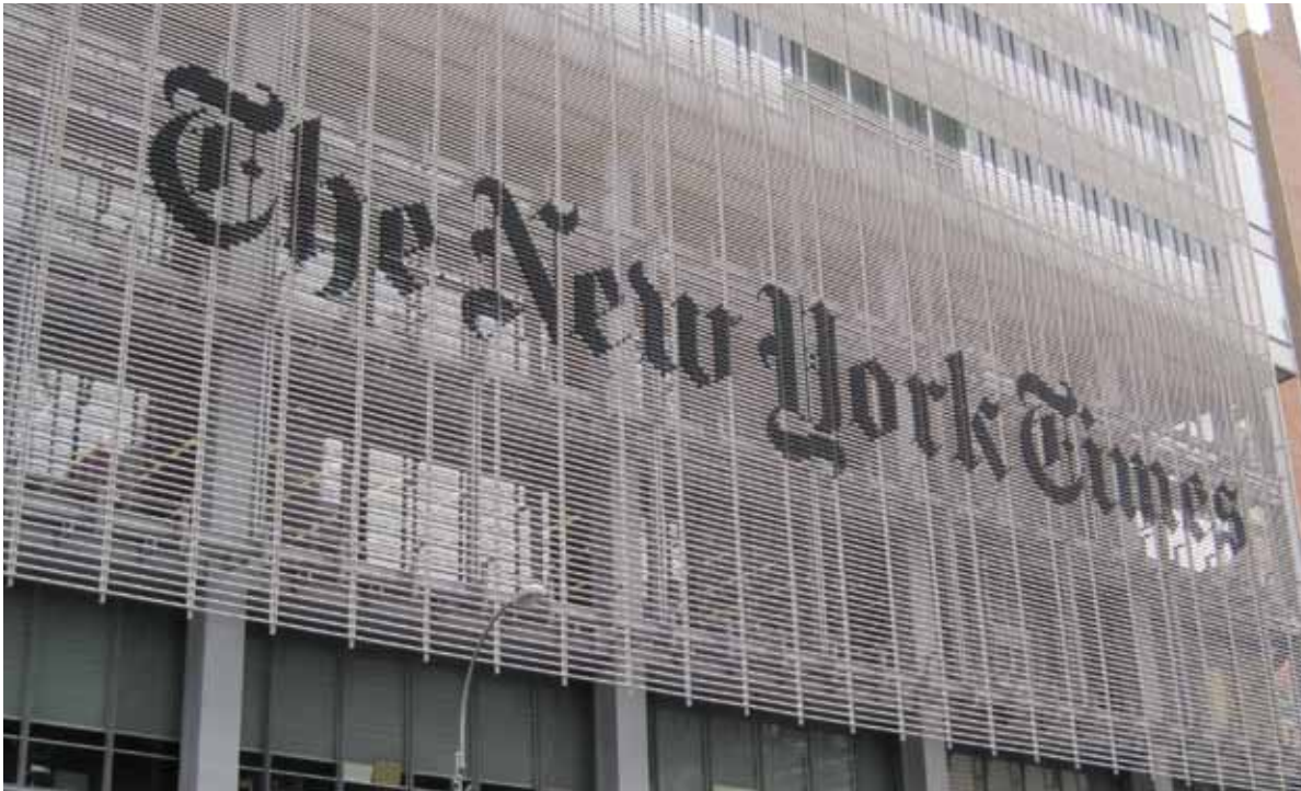
The façade of the New York Times building, by FX Fowle and Renzo Piano, is composed of ceramic rods, spaced to let occupants see out, while minimizing the extent of exposed glass. Photo: Christine Sheppard, ABC
