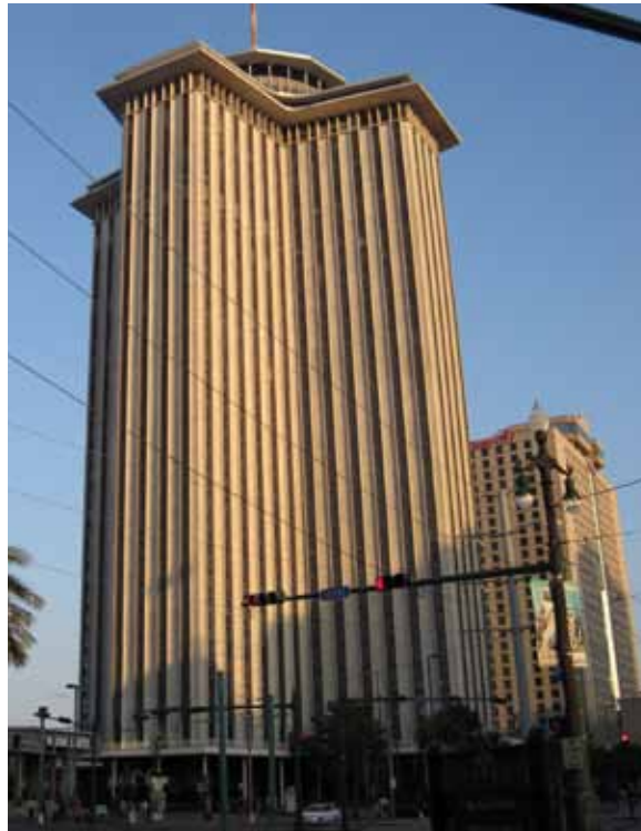
The World Trade Center of New Orleans, designed by Edward Durrell Stone, uses a simple bird-friendly strategy – almost all windows have exterior shutters. Photo: Christine Sheppard, ABC
