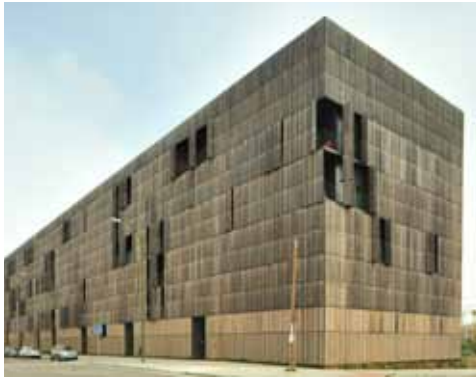
FOA made extensive use of bamboo in the design of this Madrid, Spain public housing block. Shutters are an excellent strategy for managing bird collisions as they can be closed as needed. Photo courtesy of FOA
