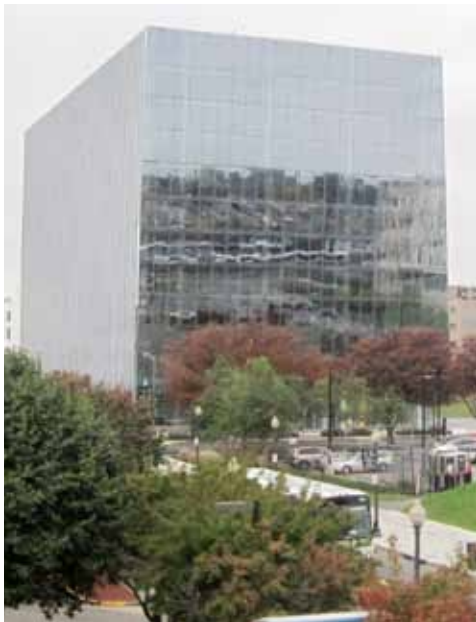
The same glass can appear transparent or highly reflective, depending on weather or time of day. Photo: Christine Sheppard, ABC
