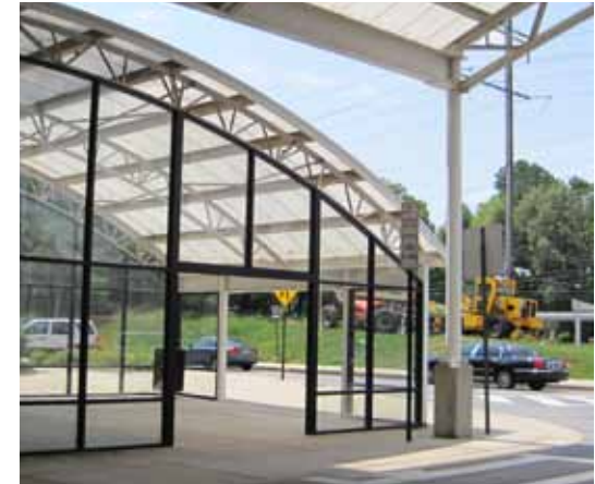
Architectural cues show people that only one panel on the face of this shelter is open; to birds, all the panels appear to be open. Photo: Christine Sheppard, ABC
