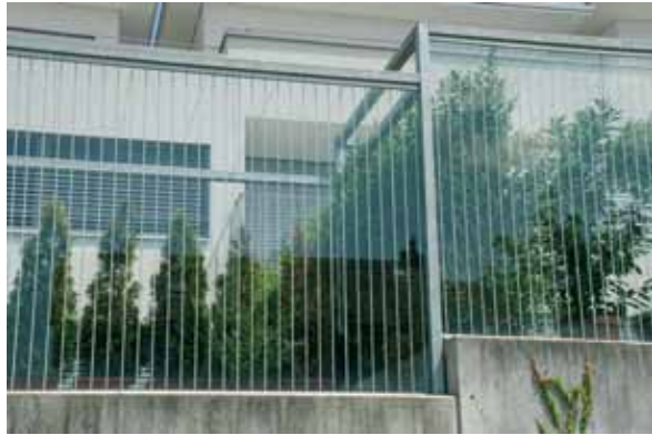
The white stripes on this glass wall are an easy way to make a very dangerous area safe for birds. Photo: Hans Schmid
