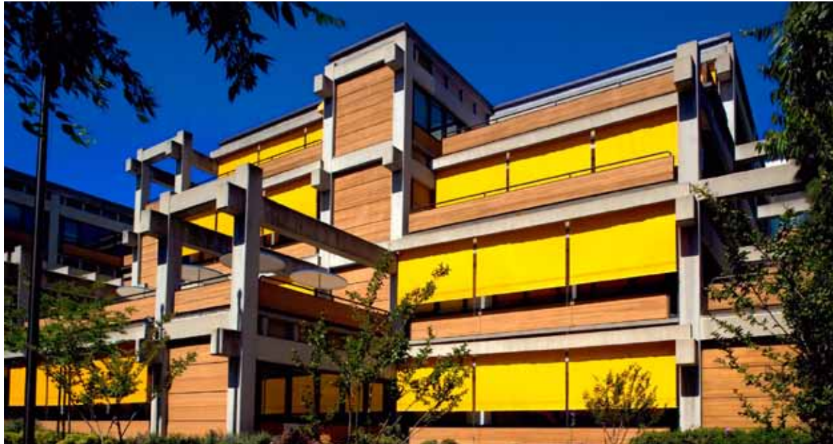
External shades, as shown here on the Batson Building in Sacramento, California, designed by Sym Van der Ryn, are a simple and flexible strategy for reducing bird collisions, as well as controlling heat and light. Photo courtesy of MechoShade
