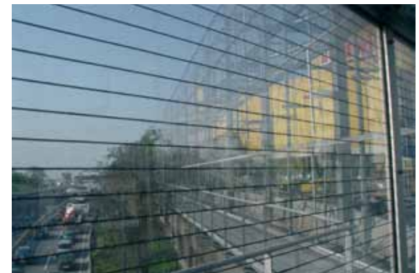
A pattern of narrow horizontal stripes has proven to be highly effective at deterring bird collisions, while covering only about 7% of the surface of the glass. Photo: Hans Schmid
