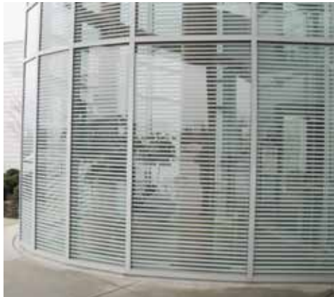
Dense stripes of internal frit on University Hospital's Twinsburg Health Center in Cleveland, by Westlake, Reed, Leskosky will overcome virtually all reflections. Photo: Christine Sheppard, ABC
